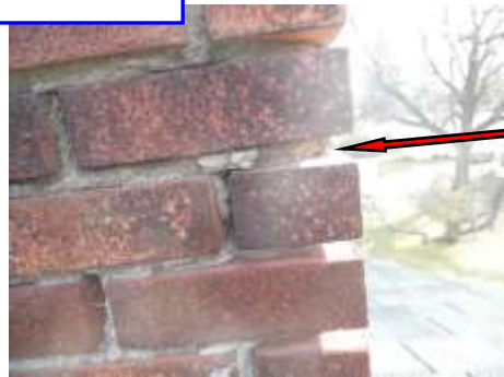
Loose mortar joints in chimney brick
