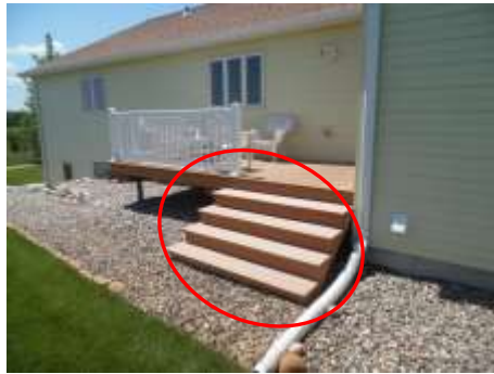
Handrail recommended on exterior steps
