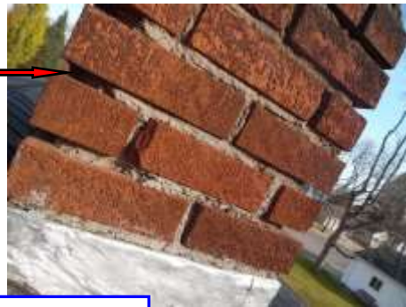
Loose mortar joints in chimney brick
