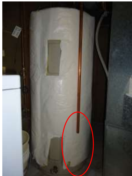
Water heater temperature relief valve extension needs to be 4"-6" off floor.
